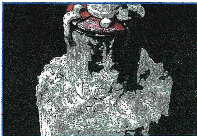
Figure 7. Bentonite cement grout seal between casings.
