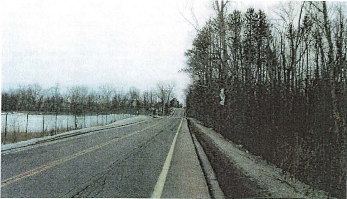
Looking northerly along Wade Road Subject at right, Airport at left
