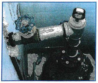
Figure 9. Completed high pressure flowing artesian well.
