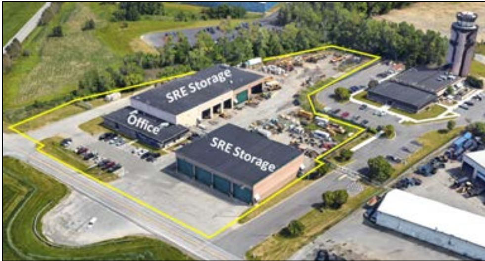
Figure 4-13 – SRE & Maintenance Buildings
