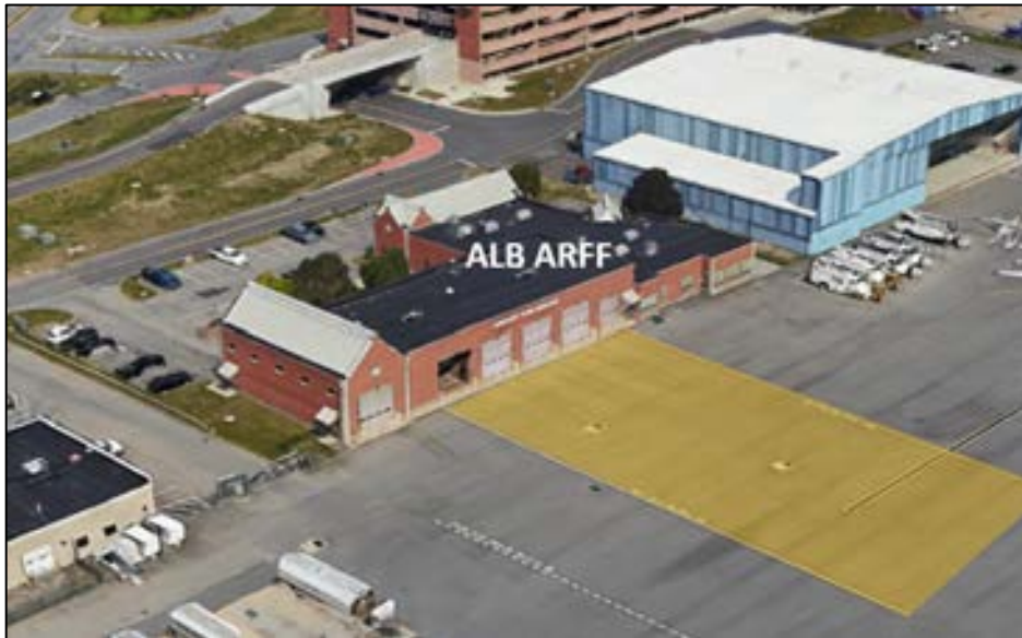
Figure 4-14 – Existing ARFF Station
