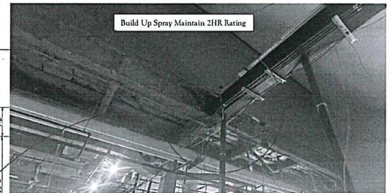
Provide 1HR rating on Roof Decking
