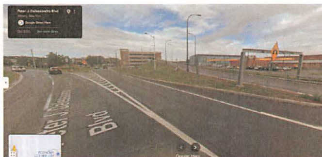
Need a sign in this location to route user to enforce Main Terminal lane
